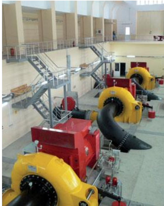
Figure 6. The machine hall with the three Francis units for SHP in Bayburt province [21].
